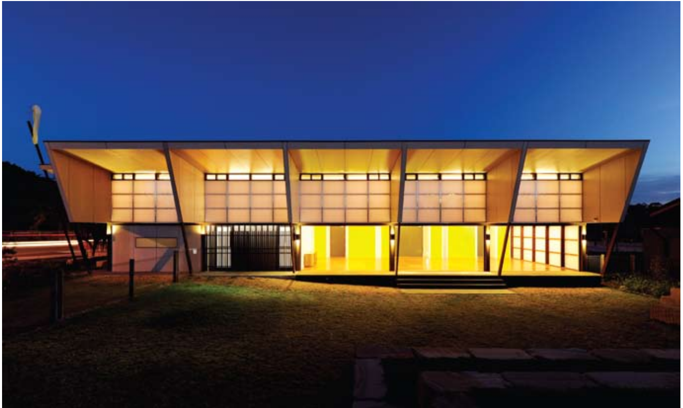
Peregian Beach Community House, awarded Building of the Year at the 2010 AIA Sunshine Coast Regional Architecture Awards. Photo: Roger D'Souza
